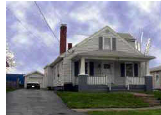
CHDO 159 Townsend St. Construction will begin shortly on this three bedroom house
